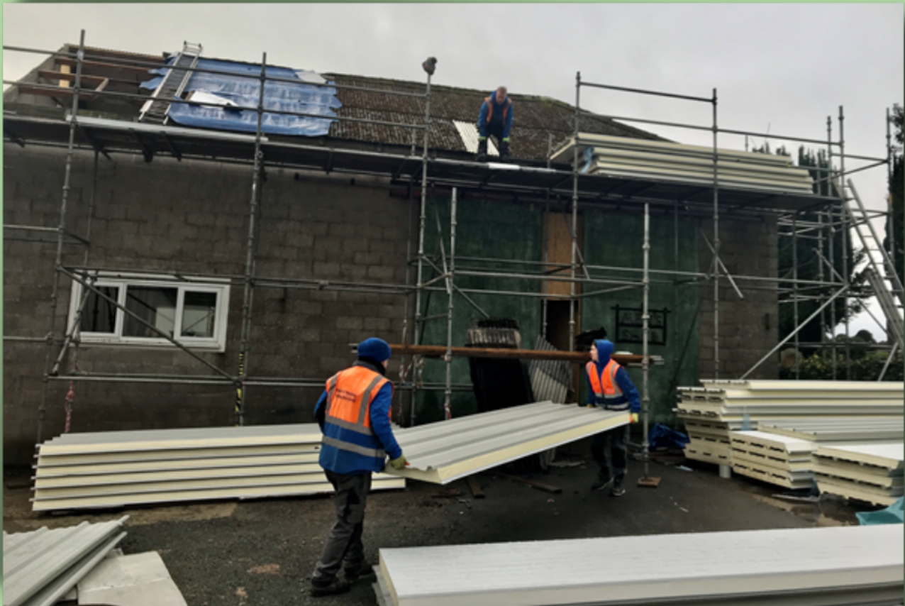
THE MEN'S SHED ROOF BEING INSTALLED
